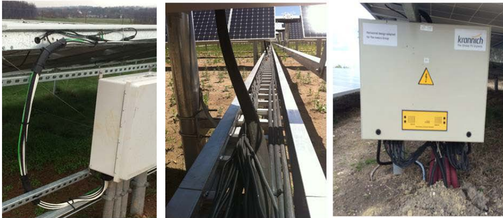
Figure 2. Maintenance of wire management systems depend on plastic wire ties and grommets, which can break or pinch wires (left); exposure to sunlight; wind and weight of ice (center); and access by chewing rodents (right). Photos by Andy Walker, NREL
