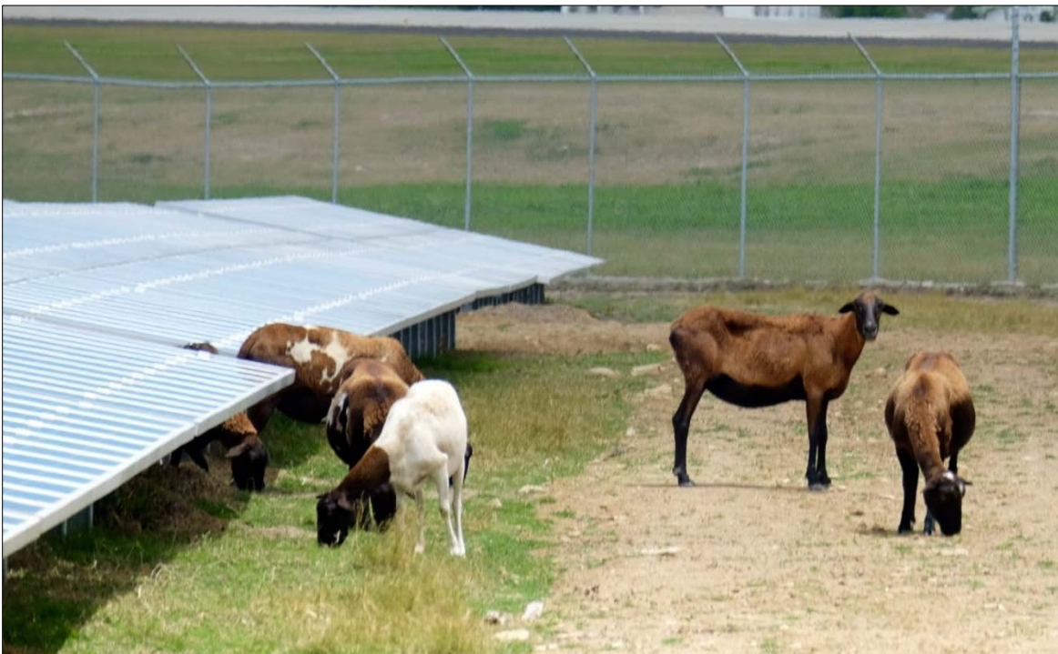
Figure 4. Sheep, but not goats or cattle, can be employed for vegetation control. Photo by Eliza Hotchkiss, NREL
