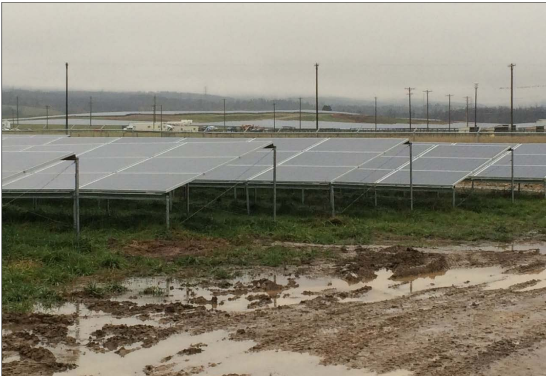
Figure 5. Drainage and storm-water run-off are difficult to improve after the PV array is installed, requiring diligence in design and construction of storm-water management systems. Photo by Andy Walker, NREL
